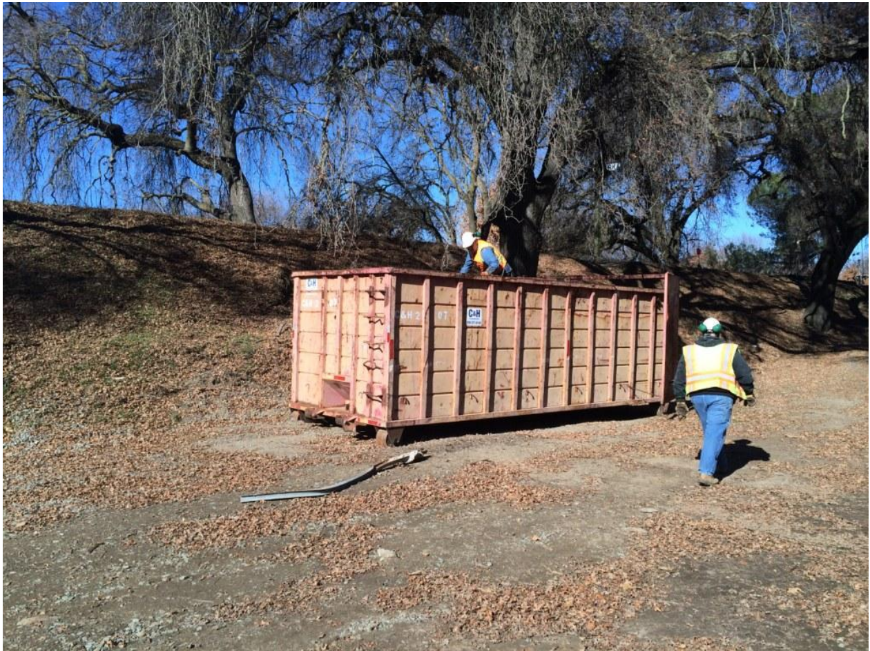
Fred organizing the dead ties in the dumpster to maximize capacity
