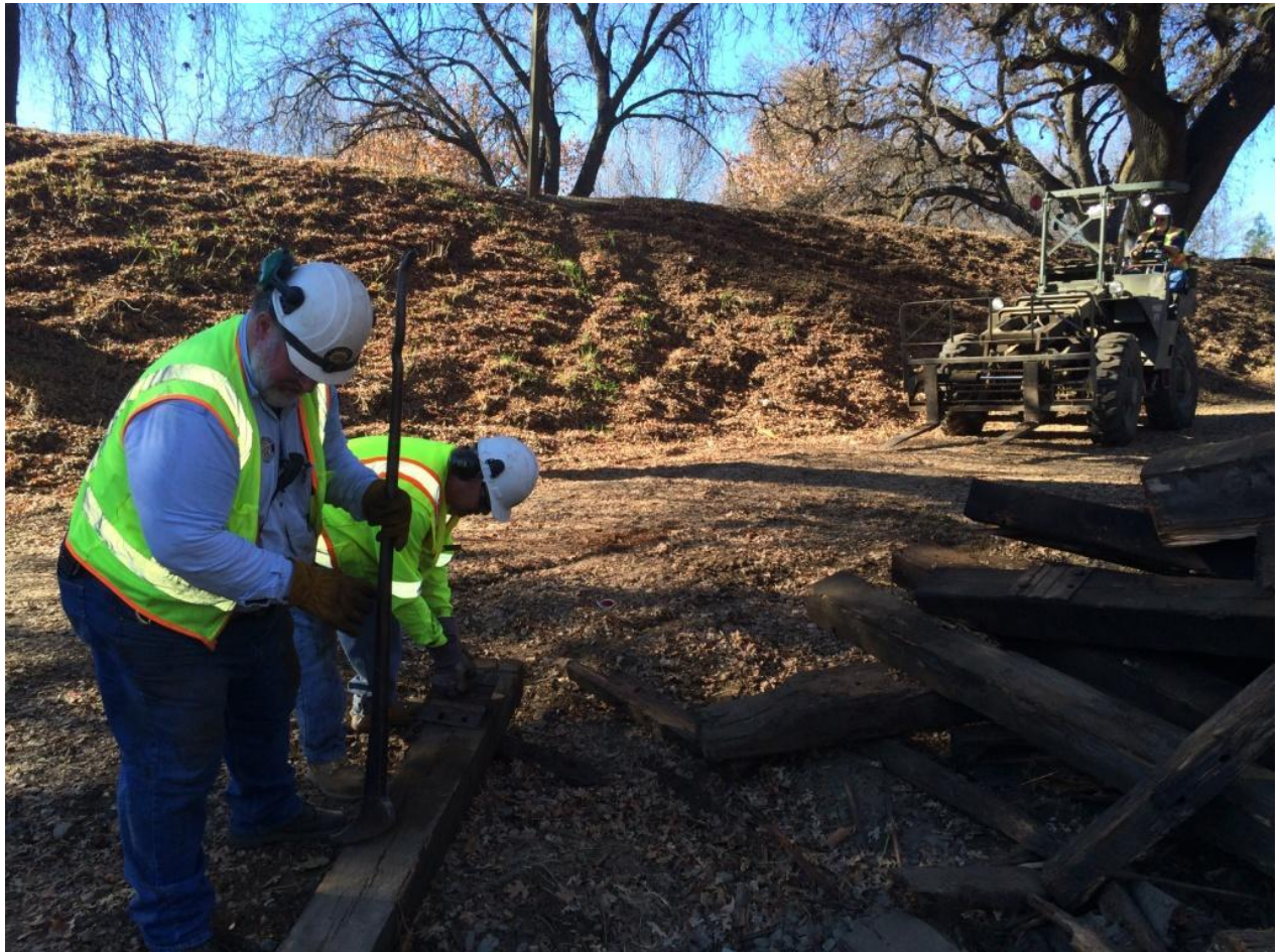
Taka and Frank remove spikes and tie-plates from the dead ties
